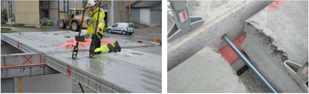
Fig. 5 Placing of a HCS with the mobile crane (left) and foam strips on top of wall nib supporting the HCS in axis C before grouting (right).
