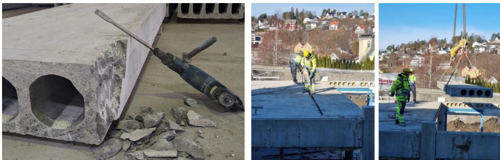
Fig. 1: Difficult removal of grouting concrete from HCS recovered from the swimming hall in Volda (Norway) (left); Right: Lifting of a HCS from a building in Lysaker (Norway) after breaking of grouting concrete with a jackhammer inducing detachment from adjacent slab (right).
