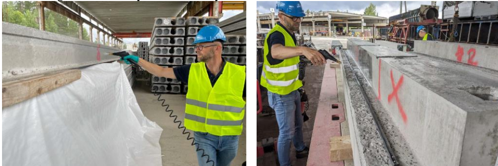
Fig. 4 Application of the adhesion-reducing products on lateral surfaces of the HCS (left) and the web of the ITB (right). Zones marked with a X specify the reference areas without products.
