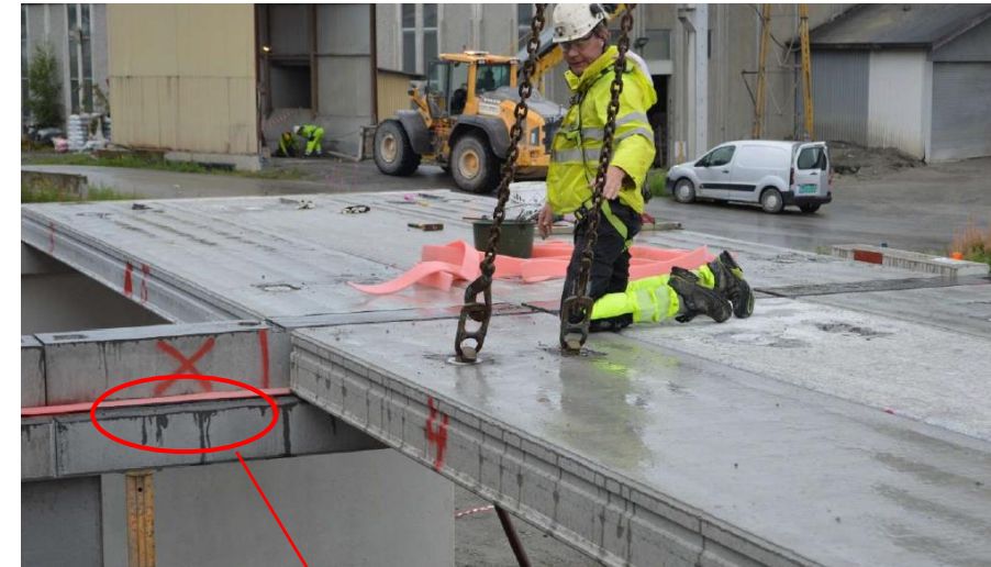
Placing of a HCS with the mobile crane
