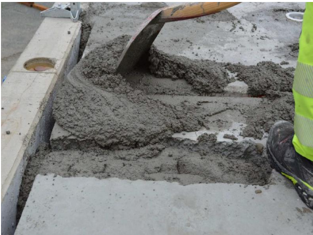
Grouting of end joints
