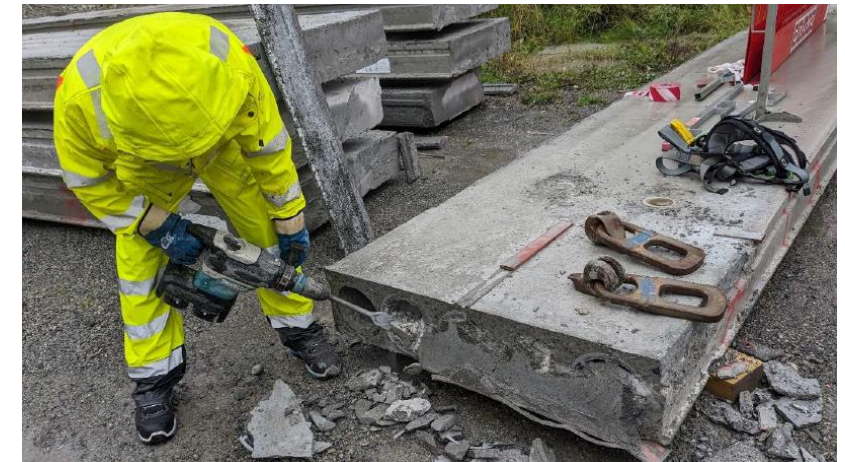
Removal from a reference area at the short end of the HCS
