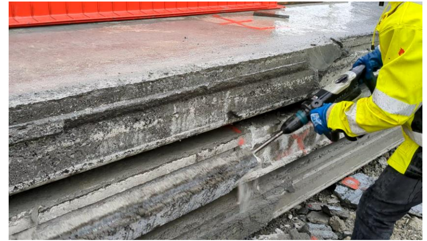
Removal of concrete from longitudinal side of HCS, where adhesion-reducing products were applied
