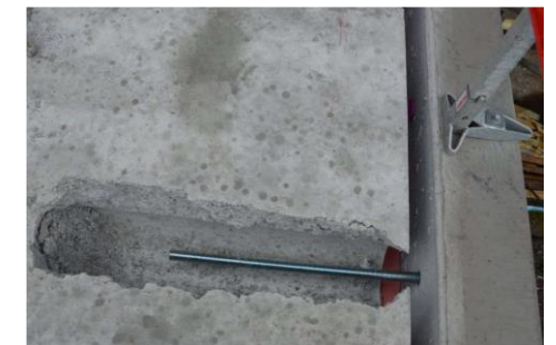
Joint between HCS and wall nib (connection III)
